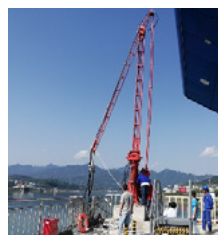
(c) Bunkering arm
