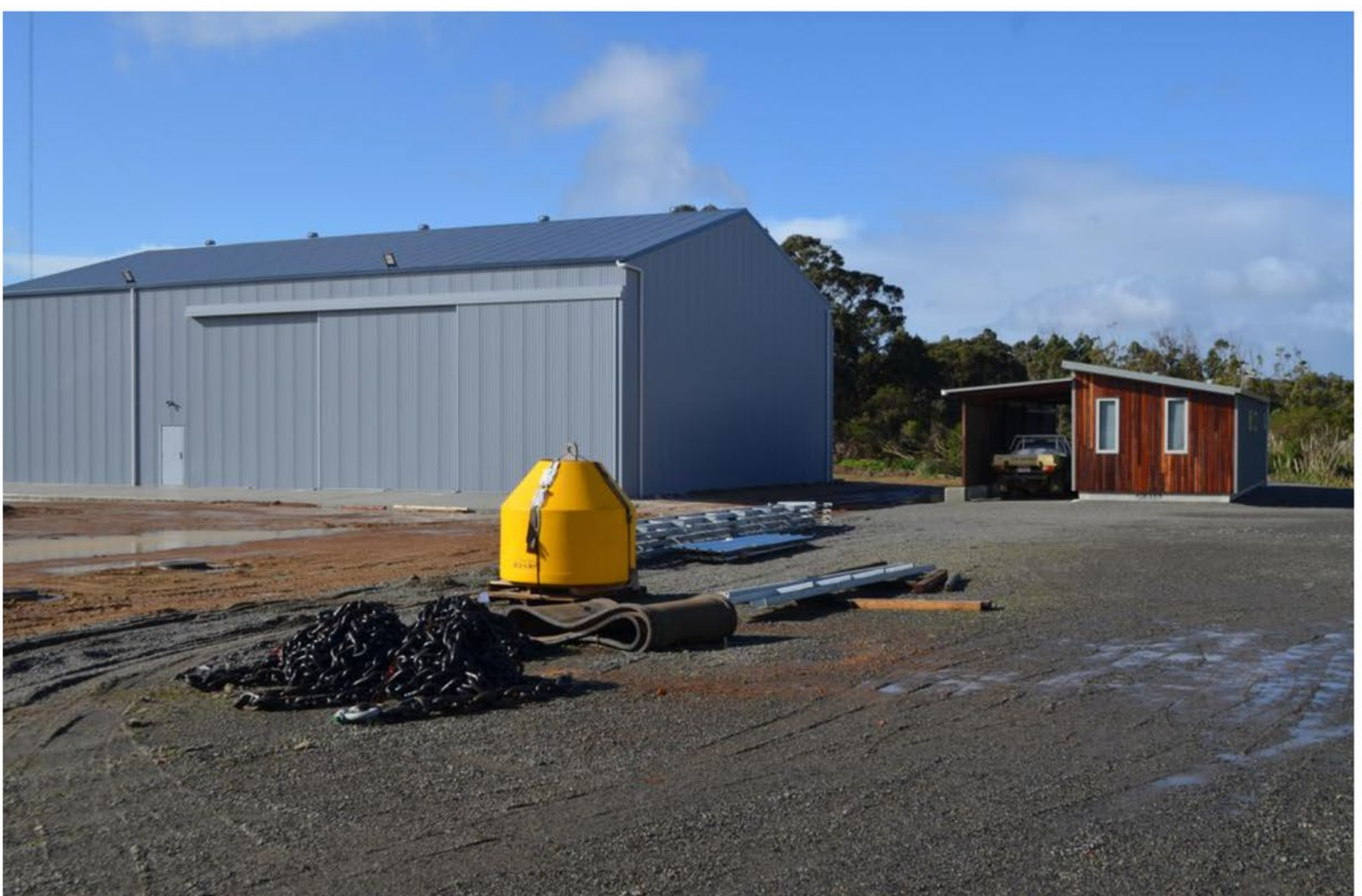
📷 Local businesses MCB Construction, RMI Engineering, Jemco Engineering, Steel Solutions WA, A1 Sandblasting, Everett Consulting, Coastal Cranes, Albany Tug Service were all involved in the device’s construction. Credit: Melissa Sheil
