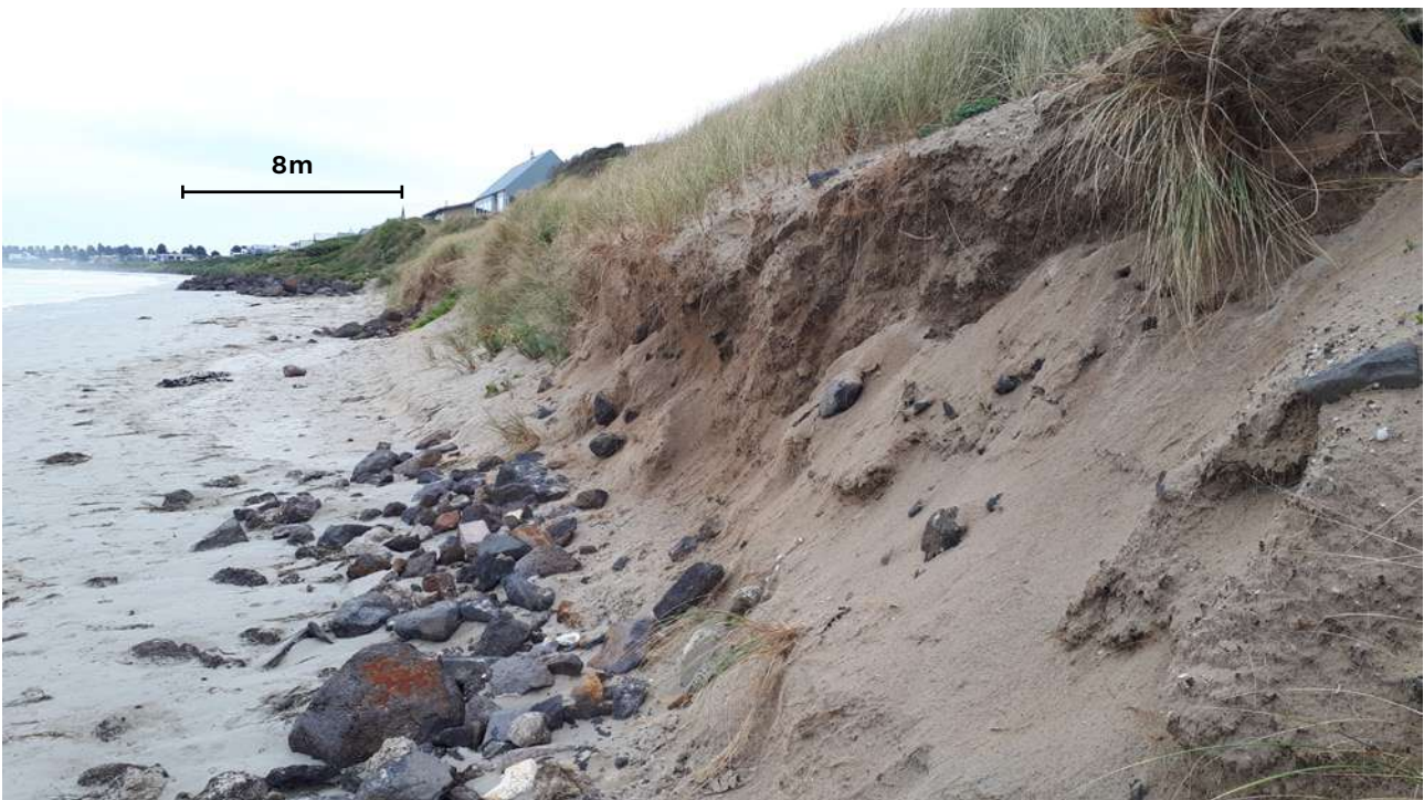
Figure 4.29. Erosion of unprotected dunes (foreground) compared to a housing zone protected by a rock revetment (middle ground). The unprotected shoreline has eroded about 8m. Photograph by Richard Manasseh.
