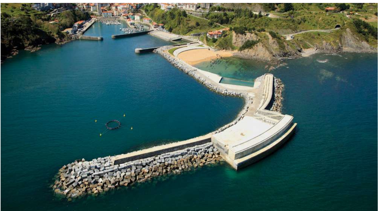
Figure 4.22. The world's only continuously operating grid-connected wave-power plant at Mutriku, Basque Country, Spain, is the longest-lived in the world and the one with the most hours of operation. (Image courtesy of www.bimep.eus ).
